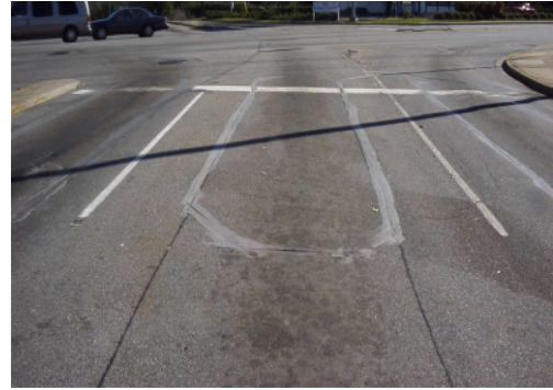
Inductive loop detection
