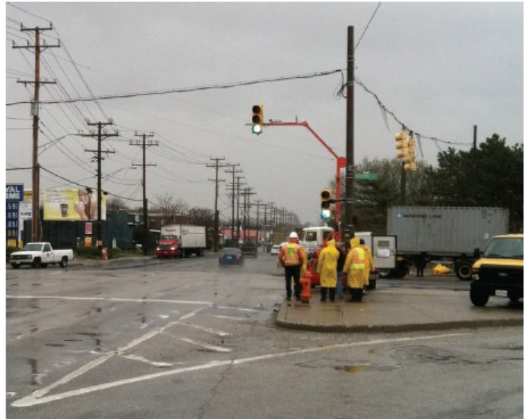
Wireless Interface System operating in Baltimore, MD.
